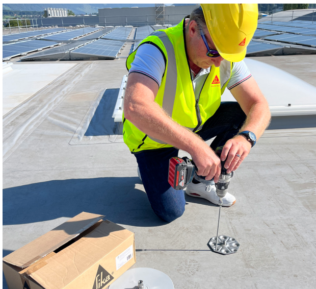
Sarnafast® Fastener SBF-6.0 or alternatively Sarnafast® Fastener SBF-6.0 with Sarnabar® Tube SBT-20.
