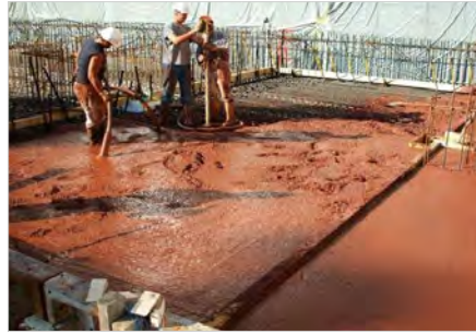
Fig. 8.16.1: The floor, walls and ceiling of this medical building were constructed with heavyweight concrete using hematite metallic aggregates to ensure full and secure radiation protection.
