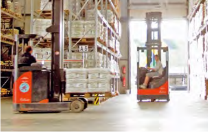
Fig. 8.7.3: Industrial flooring surfaces also experience strong abrasion due to constantly rolling and dynamic loads in the same places. Hard concrete coatings and special dispersants can enhance the grip and minimize wear.
