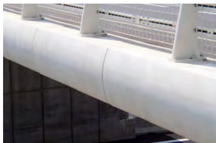
Fig. 8.9.4: Highly stressed building components such as columns and beams are made of high strength concrete. High resistance to external influences also makes high strength concrete an ideal protective coating for exposed construction elements.
